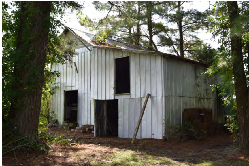
Packhouse, view to the southeast
