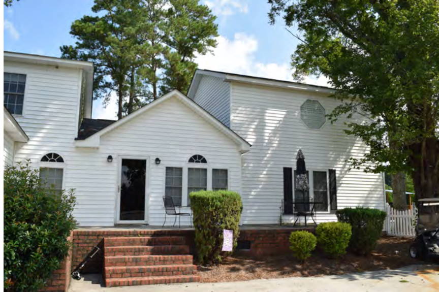
Rear additions built in 2003 and 2007, view to the north
