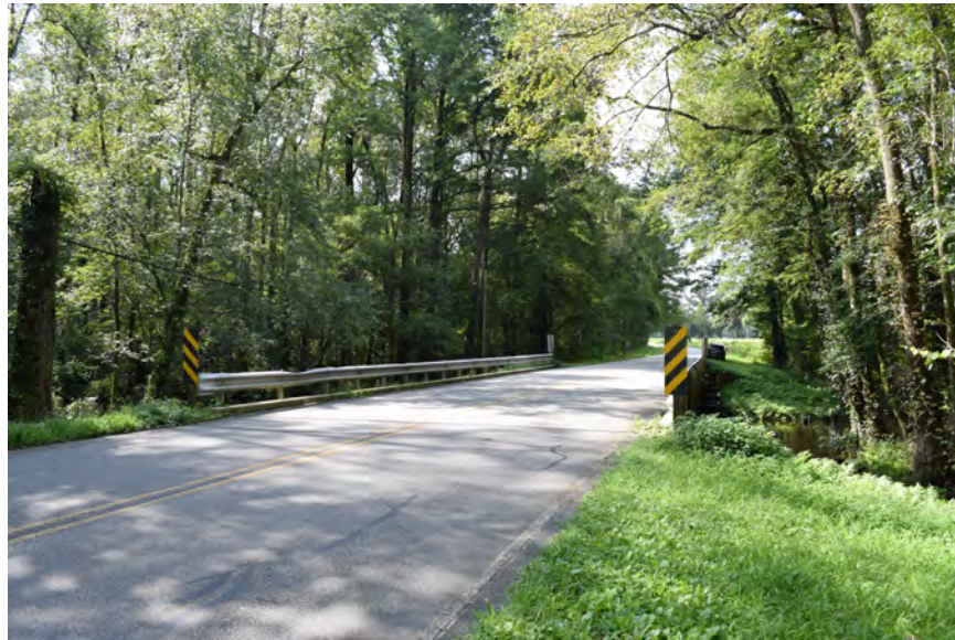
Bridge No. 6 Over Big Swamp on SR 1422 (Market Street Extension), view to the southeast
